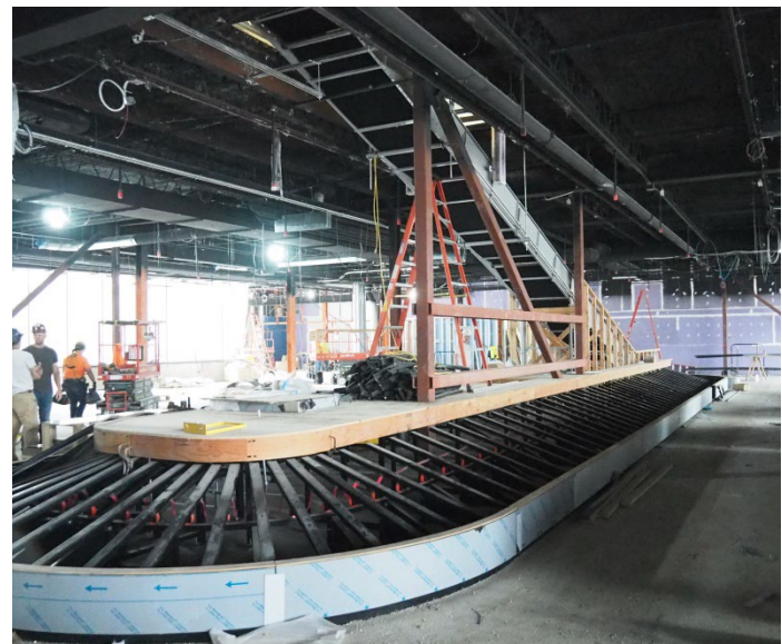
Baggage handling system carousel, under construction.
