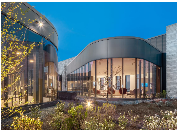
Completed TSA checkpoint and departure lounge, viewed from public patio.
