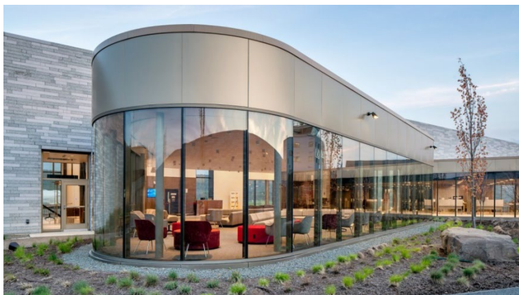
Completed departure lounge viewed from the secure courtyard.
