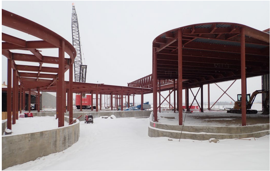
Steel erection of TSA checkpoint and departure lounge.
