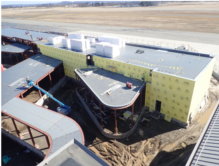
Passenger concourse structure under construction.
