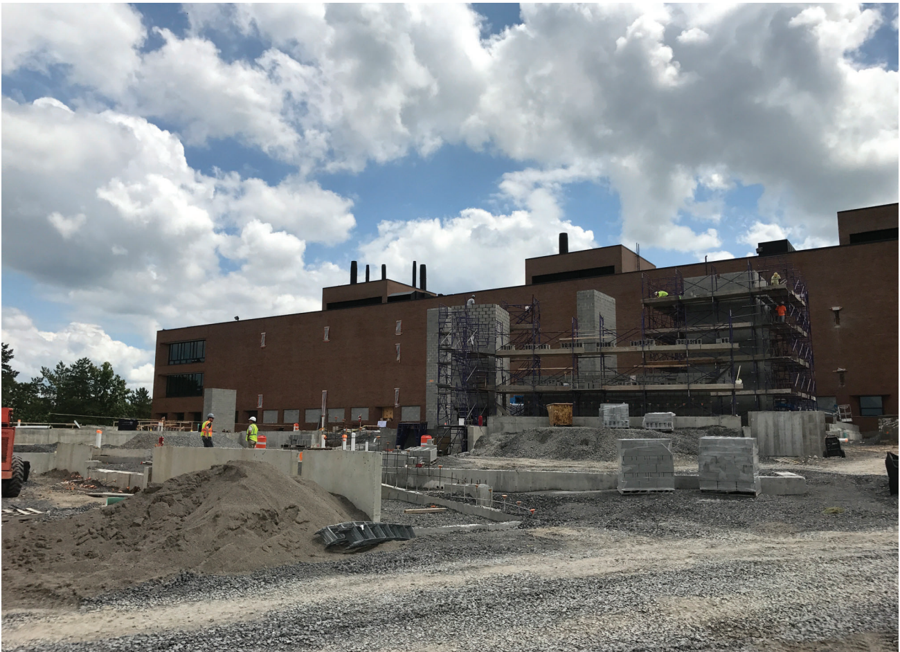
Construction-Phase Photograph of the areaways during construction
