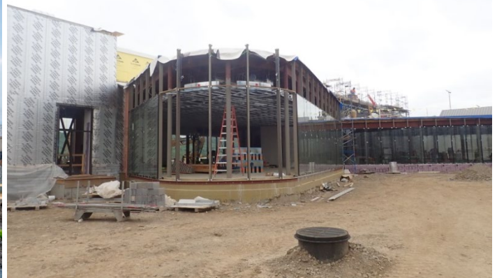
Departure lounge from the secure courtyard - structure being erected.
