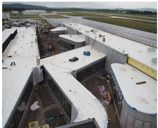
TSA checkpoint and concourse under construction.
