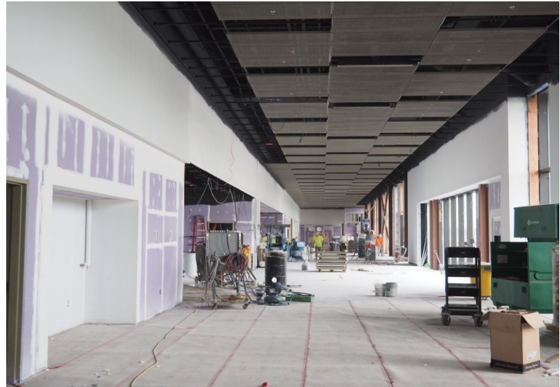
Passenger concourse as finishes are being completed.
