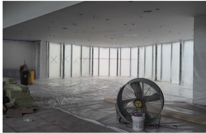
Departure lounge under construction.
