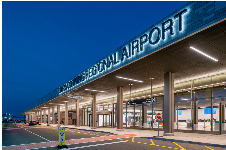
Front drive and main entrance to ticketing.
