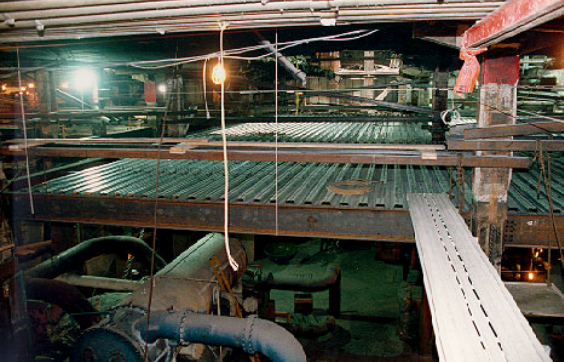
Steel Decking Being Installed Over the Refrigeration Plant
