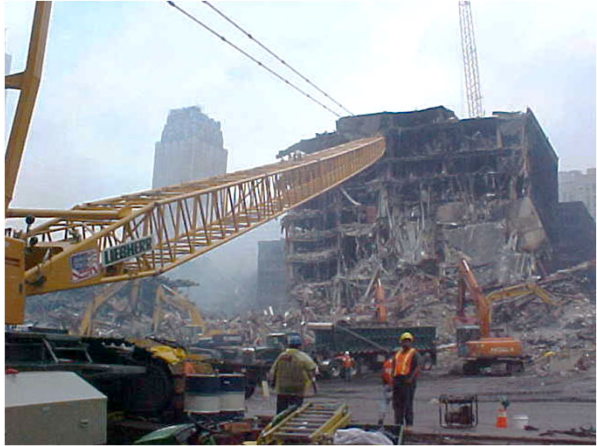
Sept 26, 2001 (Day 15): Demolition of Southeast Plaza (Bldg. 4) begins.
