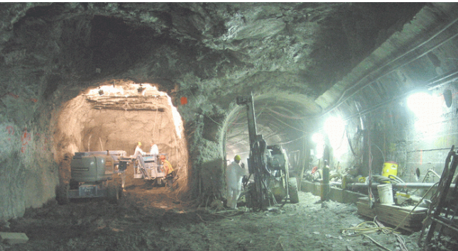
Above: Installing Rock Anchors In Newly Mined Tunnel Cross-section
