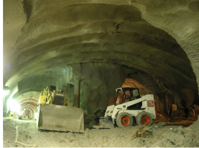
Right: Installation of Lattice Support Girders with Shotcrete
