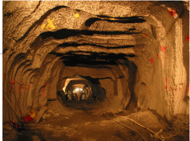
Right: Tunnel Mined in Mica Schist Rock
