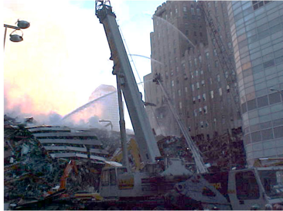
September 15, 2001 (Day four): World Trade Center Building 7 (lower left) still burning.
